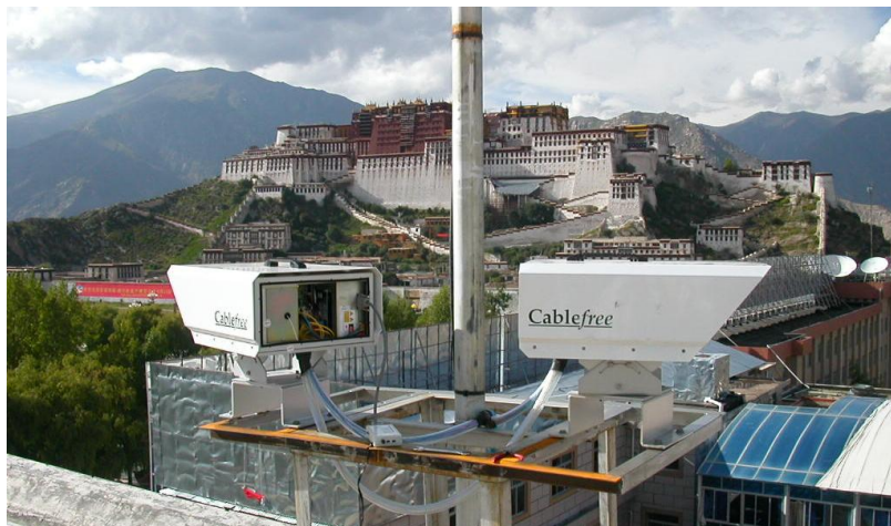
Last-mile application for China Unicom in Tibet. Shown here is a repeater site to provide non-line-of-sight connection from fibre ring to end-user site. Potala palace features in background.
