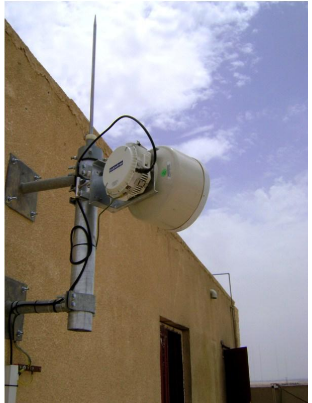
CableFree Microwave links used in Last Mile applications in the Middle East
