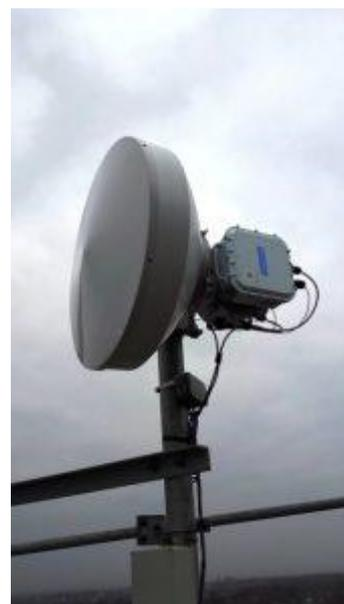
CableFree MMW link installed with 2+0 configuration
